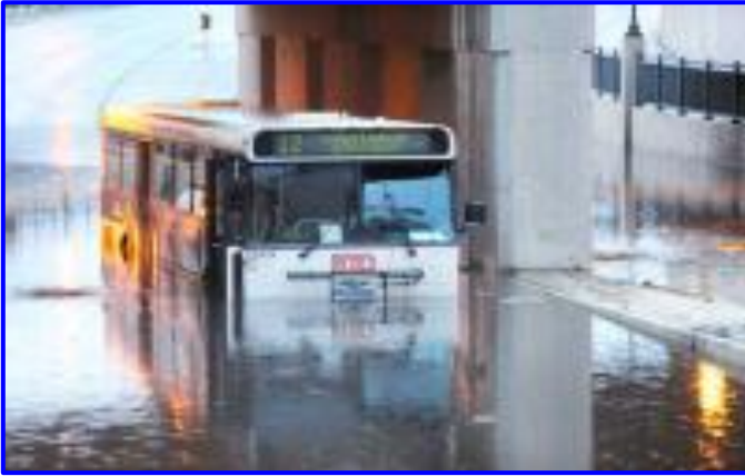
Figure 2: Urban Flooding in Denver on 7/7/11.
