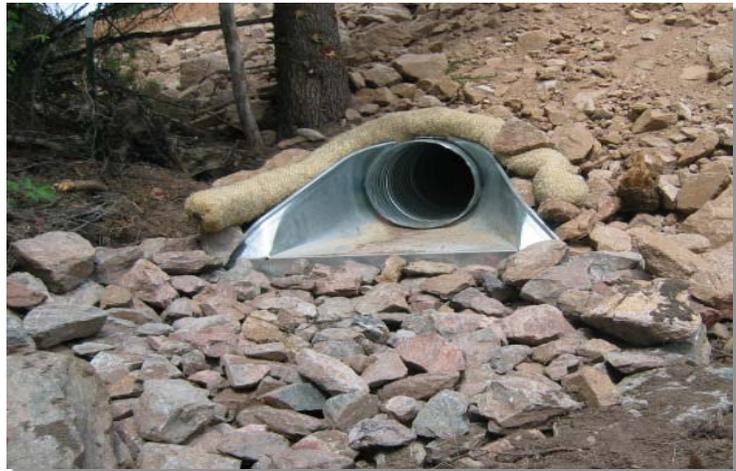
**Photograph TOP-1.** Riprap outlet protection.
