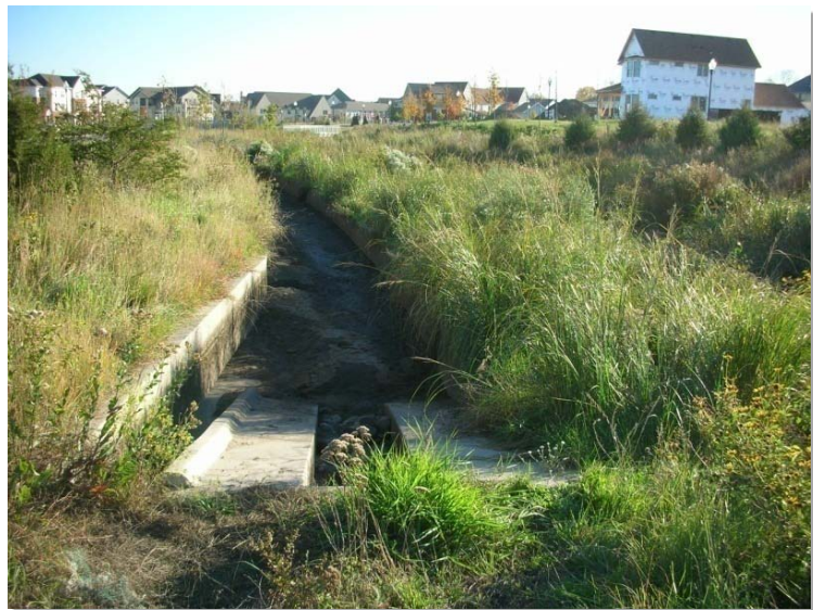
Photograph GB-4. Maintenance access is provided via the ramp located at the end of the basin. Photo courtesy of Bill Wenk.
