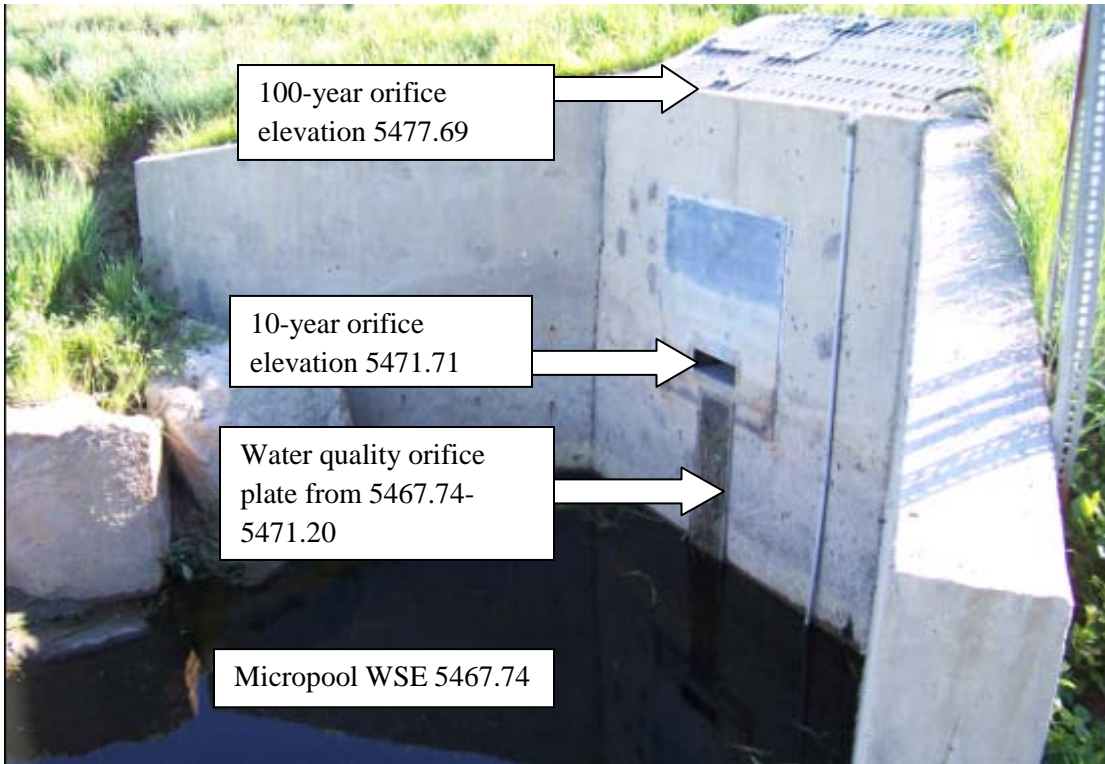
Photograph 3. Outlet structure with micropool
