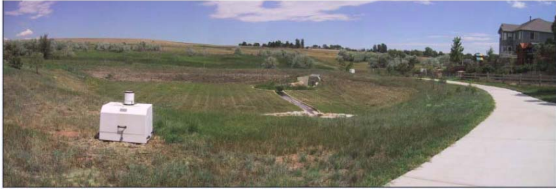
Photograph 1. Grant Ranch EDB with inflow sampler box shown in the foreground.
